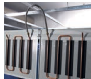
fig. 2.9 Inspectionability of GK PSV radiant ceiling – active and passive panels suspend by wires
