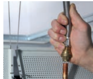
3. The water system connections come next: the panels part of the same circuit are connected one to the other, while the first and last panel of the series are connected to their distribution manifold, one for delivery, the other for return.
