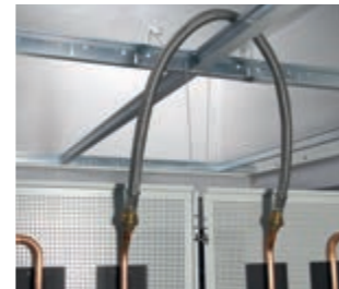
4. Connection detail for two adjoining panels
