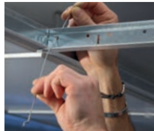
1. The PGK metal wires are fitted into the corresponding support holes
